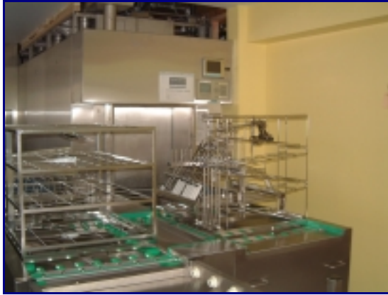
New sectional washer/ disinfectors. Capable of cleaning up to 45 surgical sets per hour
